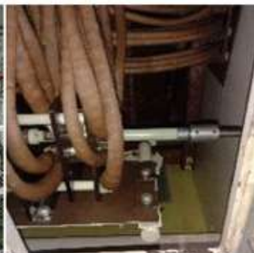
Tap switch handle replacement of 31.5MVA
