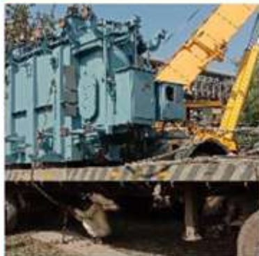
Shifting of transformer
