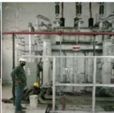
Heat exchanger service of Furnace Trafo.
